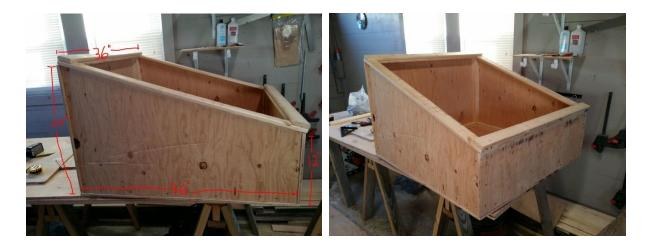
The plans are for the thicker plywood build without the framing so you can build it faster and easier. If you decide to frame it you can just measure the lengths to fit in the seams after building the box as I did.
