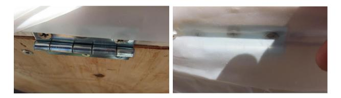
I screwed on the hinges under the plastic and connected the door to the unit. I then stapled the end plastic over the hinges and let it extend a couple inches to overlap the gap. This helps keeps the heat the in the box as heat rises and could escape if it was an open gap.
