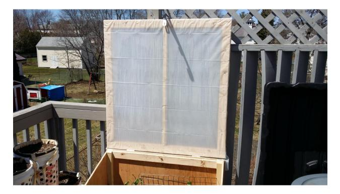
Once your square is complete simply cover it with plastic on both sides and staple it onto your frame. I allowed the plastic to overlap a bit so I could staple in on the edges as well so there was not exposed wood showing.
